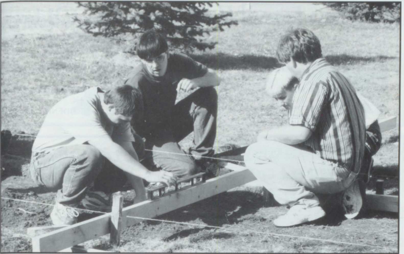
Above: Shop teacher Brian Jorgensen helps JayTee Sealey, Dan Soesbe, and T.J. Wieckum level the forms for the new sidewalk which is located on the westside of the elementary building. Left: School counselor Susen Schirmer talks to Erin Bolton about career choices.
